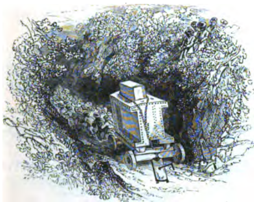
BOILER ASCENDING THE 'HILL OF DIFFICULTY.'
